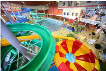
A large, heated body of water continuously evaporates moisture into the air. The more activity in a pool, the more evaporation.
